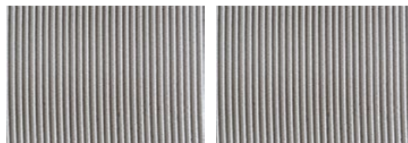
OK Spreading on substrate and tile in same direction
