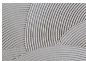
NO Incorrect application
