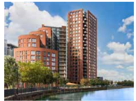
Galliard Homes, Orchard Wharf London, UK
