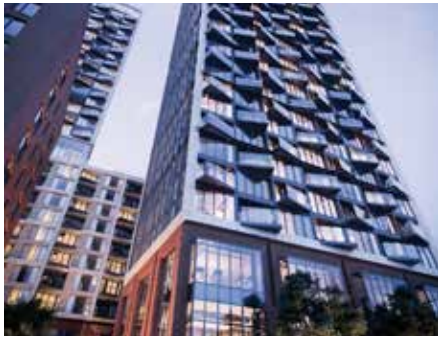
Portal West, London, UK
