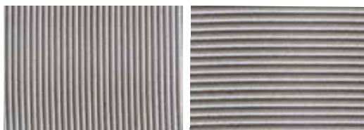
NO Spreading on substrate perpendicular to spreading on tile
