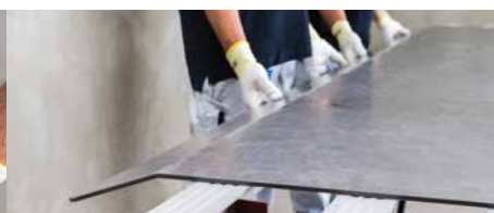
5. Snapping the slab
